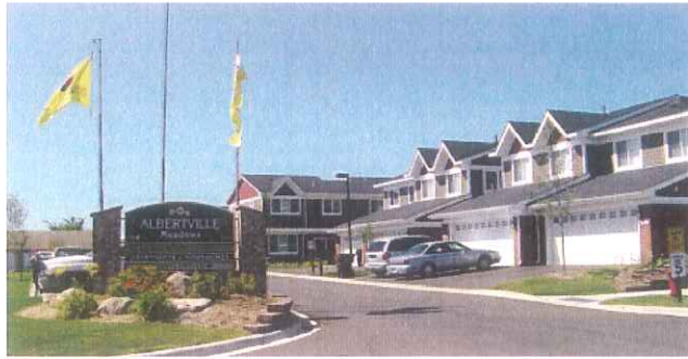
Albertville Meadows Townhomes features 37 affordable housing units, including four for formerly homeless families, in Albertville, Minn. The $8.4 million project is one of Dominion's latest developments.
